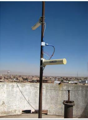
Data is transferred via YAGIs or parabolic antennas to be uploaded to internet
